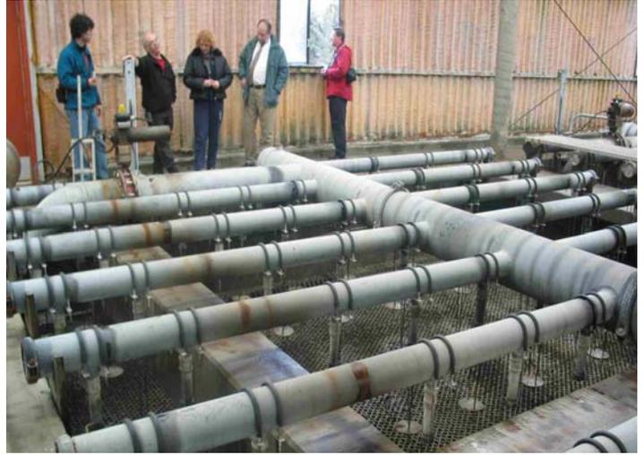
*Figure 18. (Right) Wastewater is sprayed onto a grill coated with bacteria that absorb dissolved organic matter and trap particles.*
